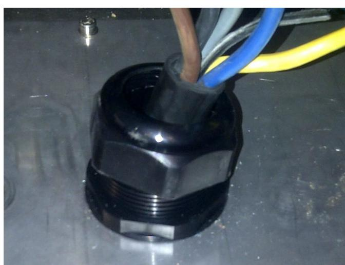
1. Slide the cable gland(s) over the cable(s).
