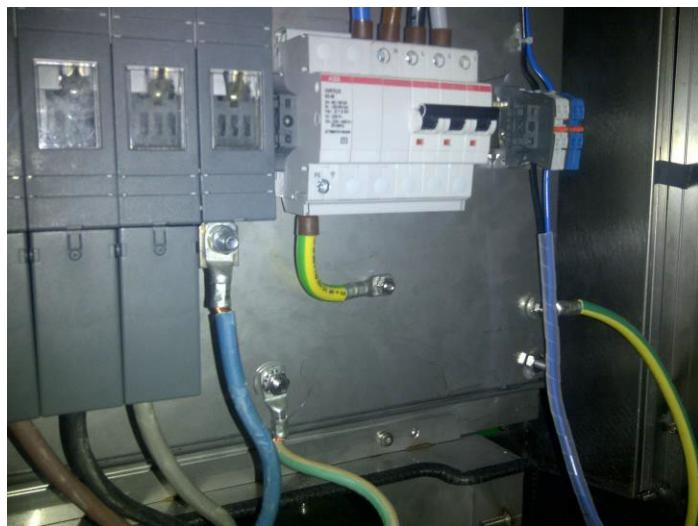
1. Cut the PE wire of the power cable to the correct length to reach the PE connector.
