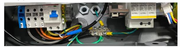
12. Tighten the bolts. The advised torque value is 2.9Nm.
