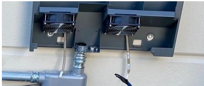
Conduit Install shown as a comparison
