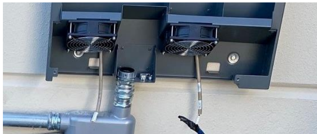
Conduit Install shown as a comparison
