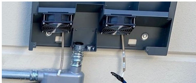
Conduit Install shown as a comparison
